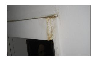
A gap in the kitchen paneling allows air to escape
