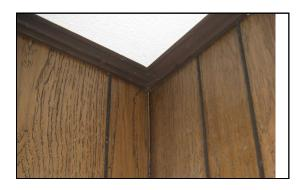
Window and door trim throughout the house are allowing significant air leakage. Pulling the trim off and filling with a two-part foam designed for doors and windows is recommended.
