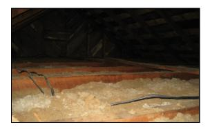
The Attic hatch on the second floor, and the one in the southern addition should both be air sealed and insulated up to R38. This can be done either with fiberglass batt or rigid insulating sheathing.
